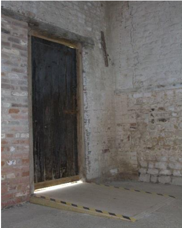
Access Ramp in East Barn
