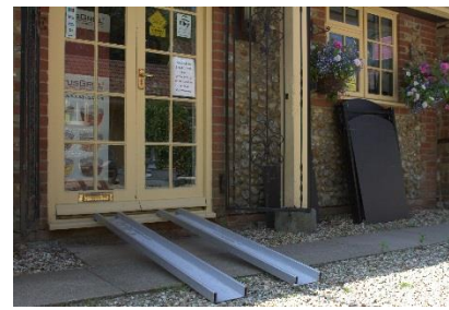
Access Ramp to Shops
